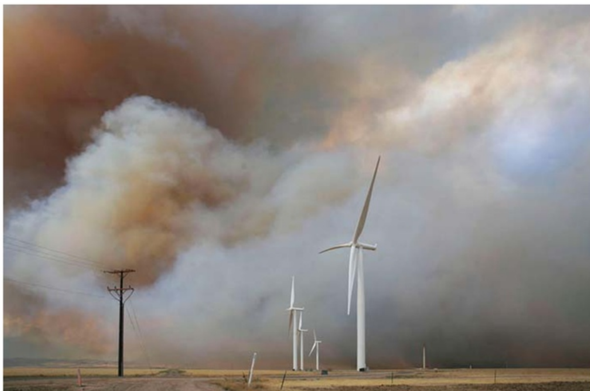
Utility poles and wind turbines in the path of an approaching wildfire. Photo by POWER Engineers.
